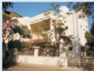
Co-ordinating Office, Ahmedabad
